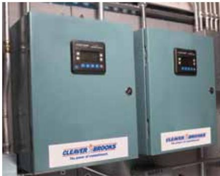
The 3" HMI provides the Operator access to the Control screen, alarm history screen, and monitor I/O screen. Secured screens are provided for loop tuning and for initial system setup.
