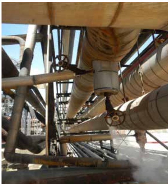
▲ Figure 7. A 400-ft section of a 24-in. steam main experienced 7 ft of movement (as evidenced by the angled horizontal and vertical piping on the left side of the photo) due to an estimated water mass exceeding 3,000 lb.
