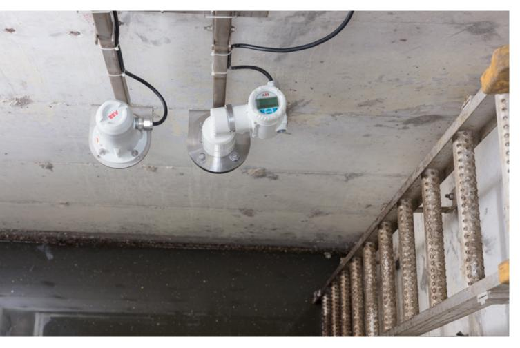
01 ABB laser level transmitters used in municipal wells to measure wastewater level. Lasers enable level monitoring measurement for various dry bulk solids and liquids stored in vessels. They can measure through narrow gaps and down to the bottom of vessels. They work in all types of storage vessels, including silos, tanks, feed chutes, bunkers, and hoppers.
