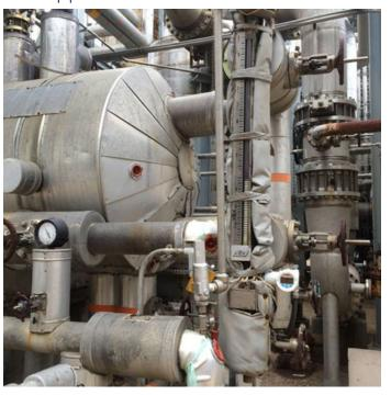
The customer has a critical ammonia ( $NH_3$ ) vaporizer unit used for NOx control. The application had an existing K-TEK KM26 and transmitter installed on it since 1998.
