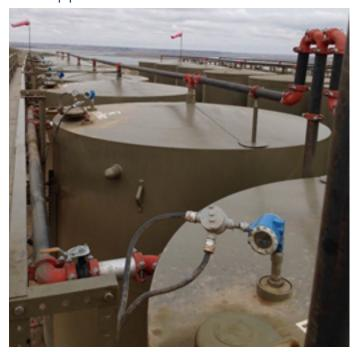
The customer is an upstream oil and condensate producer and is interested in a reliable level and interface measurement in his collection vessels.
