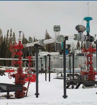
Figure 2: The well pads experience freezing temperatures for half the year, so many well pad functions are contained in heated sheds (background), one for each wellhead.
